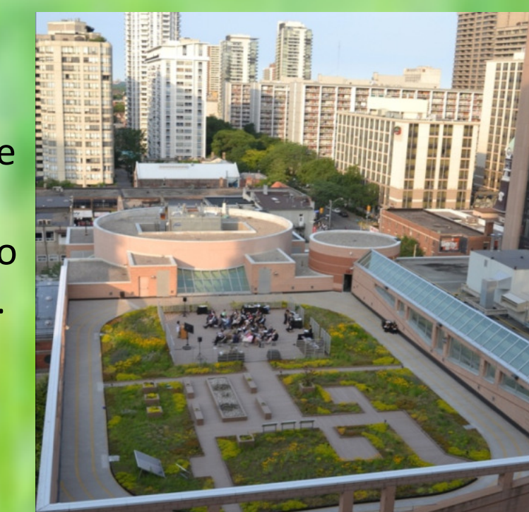
Figure 7: View of Metro Canada, YMCA, Intensive Green Roof, on institutional building, part of the Eco-Roof Incentive Program Case Study.
