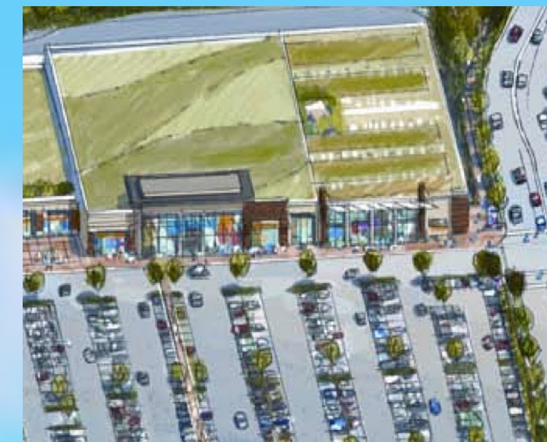
Figure 6: Green Roof on Walmart store, City of Port Coquitlam, B. C.
