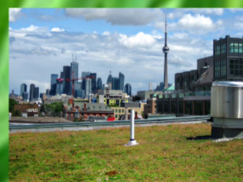
Figure 3: View of Extensive Green Roof at Gladstone Hotel (Toronto, ON), on commercial building, part of the Eco-Roof Incentive Program Case Study.
