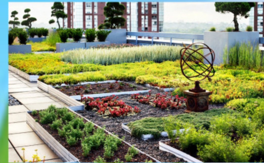
Figure 1: View of Extensive Green Roof at ESRI Canada's commercial building, part of the Eco-Roof Incentive Program Case Study.
